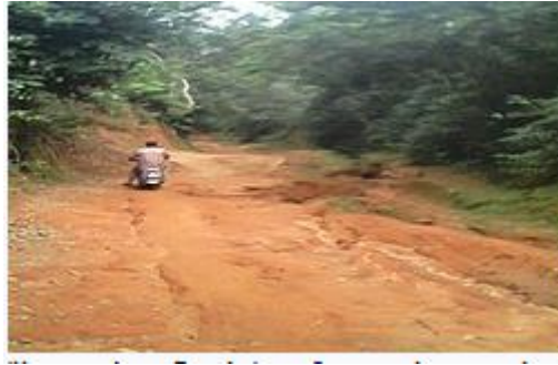
Figure 1: Untarred historic “Umuezukwe Road”, a flood channel to pollution of Njaba River, Umuezukwe, Awo-omamma
